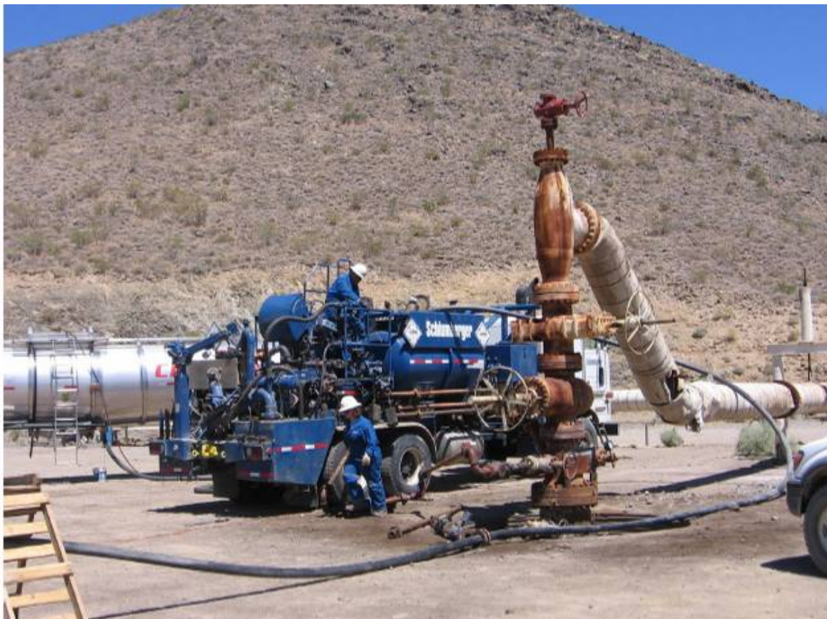
Figure 10 - Installation of a pumping unit for injection of chemical compounds at Coso geothermal field (photo P. Rose, EGI, Univ. of Utah).
