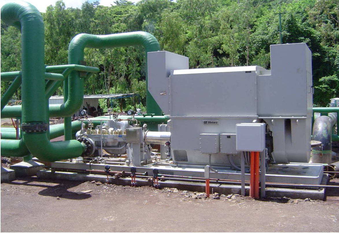
Figure 12 - View of injection pumping system at Berlin Geothermal field, in El Salvador.
