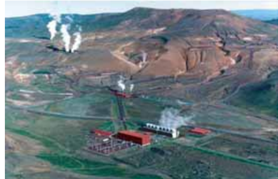
Geothermal site and plant at Krafla (Iceland).
