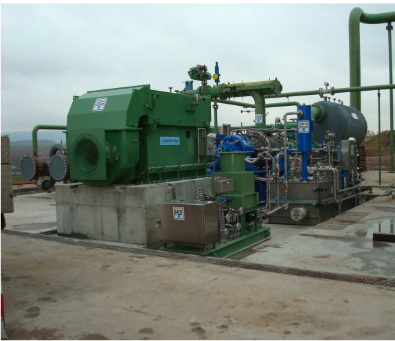
Fig. 13. Generator (foreground) aligned with the turbine.
