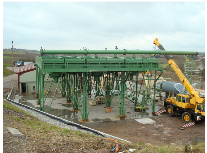
Fig. 11. Installation of the air cooling system
