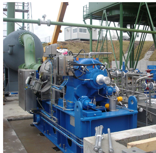
Fig. 12. The turbine being installed.
