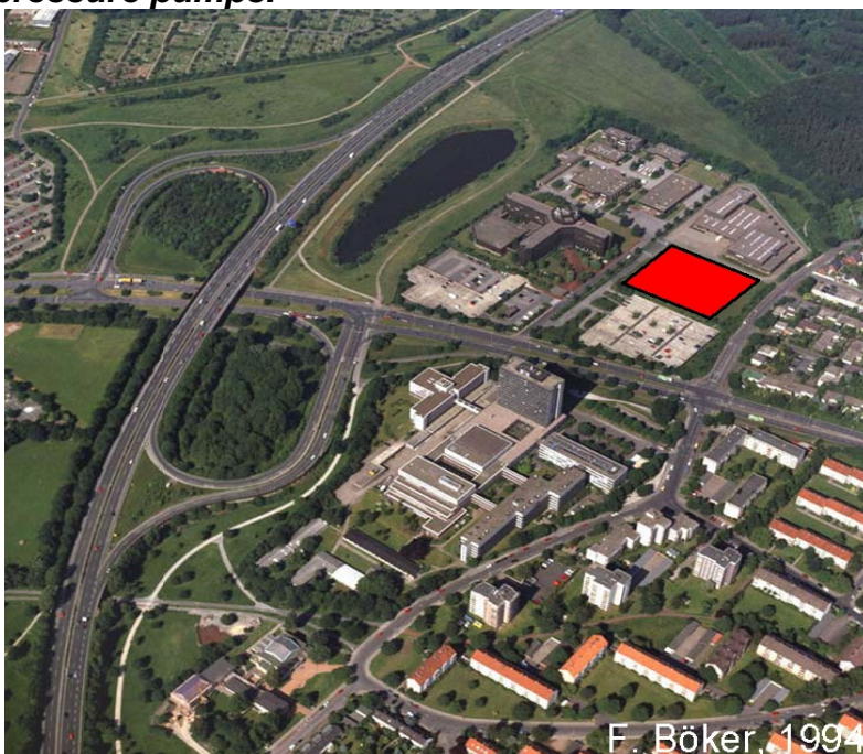
Figure 2 : Hannover test site (red area) next to the GEOZENTRUM Hannover.
