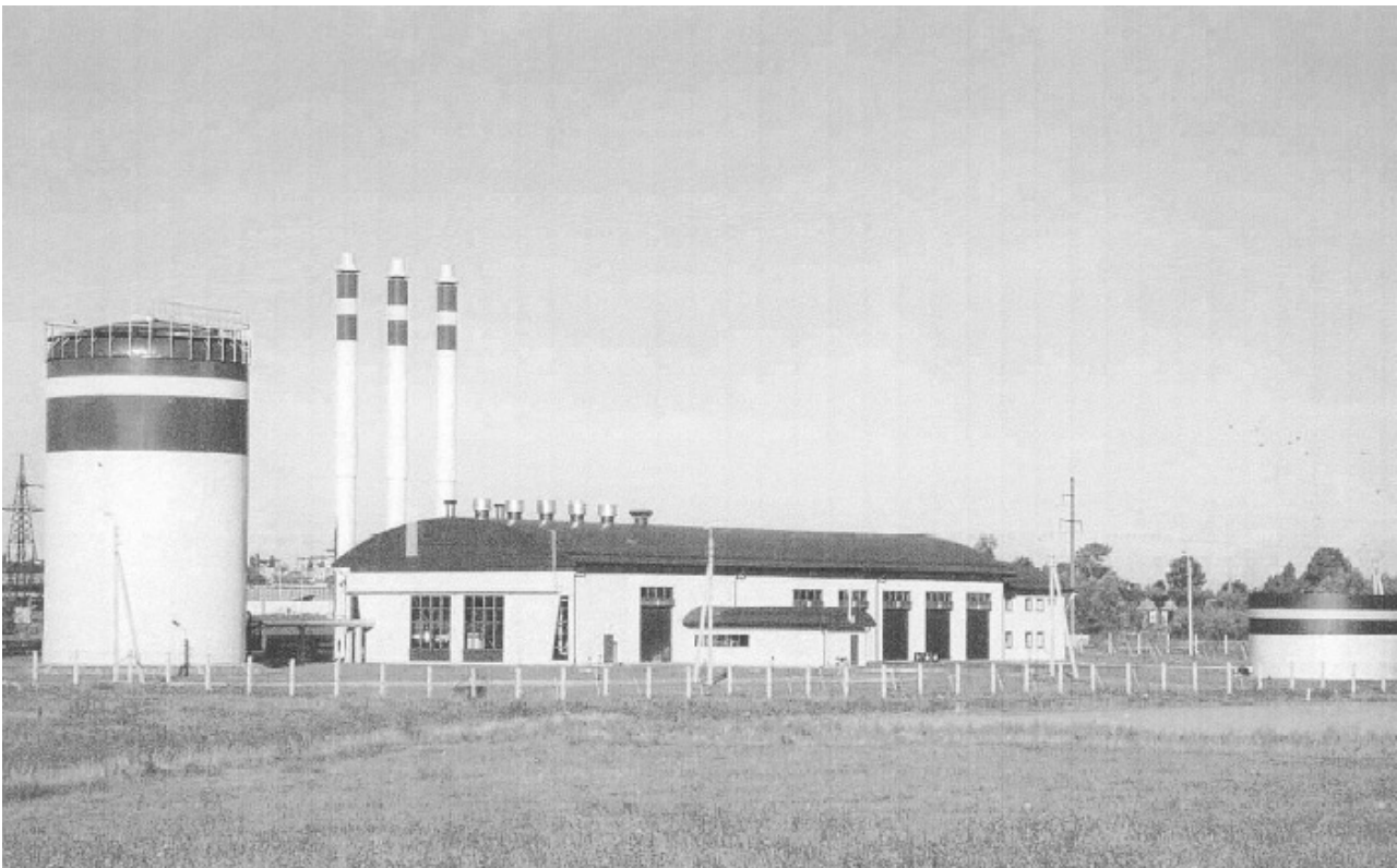
Figure 1 : View of Klaipeda Geothermal Demonstration Plant
