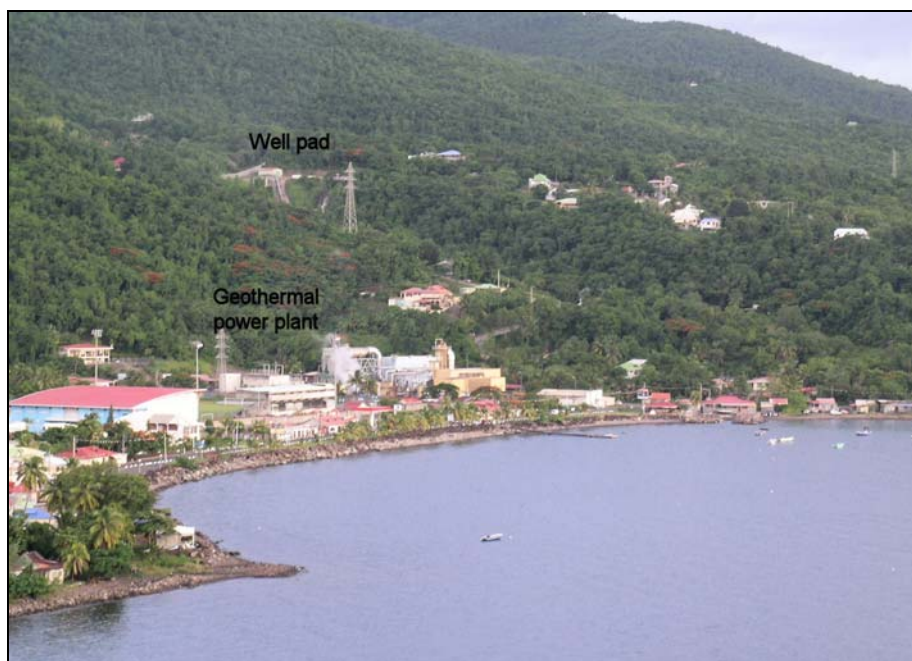
Photo of the Bouillante geothermal power plant located within the City and close to the seaside. the distance between the plant and the well pad is about 600 m.
