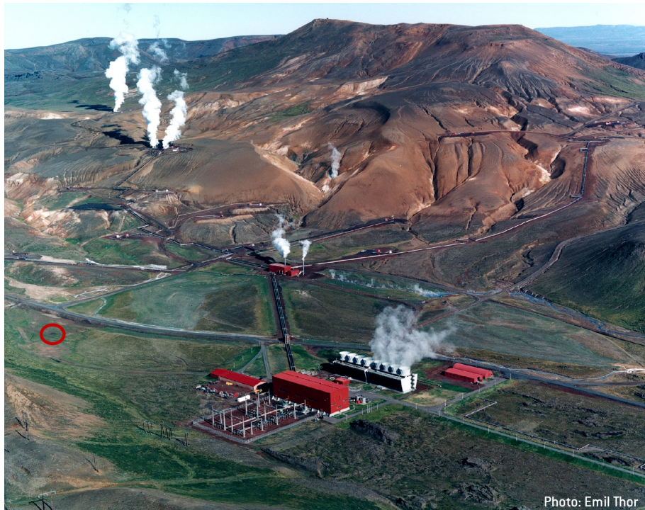
A view to the Krafla Central Volcano. A 60 MW power plant is seen in the foreground. The red circle denotes the potential IDDP drillsite.
