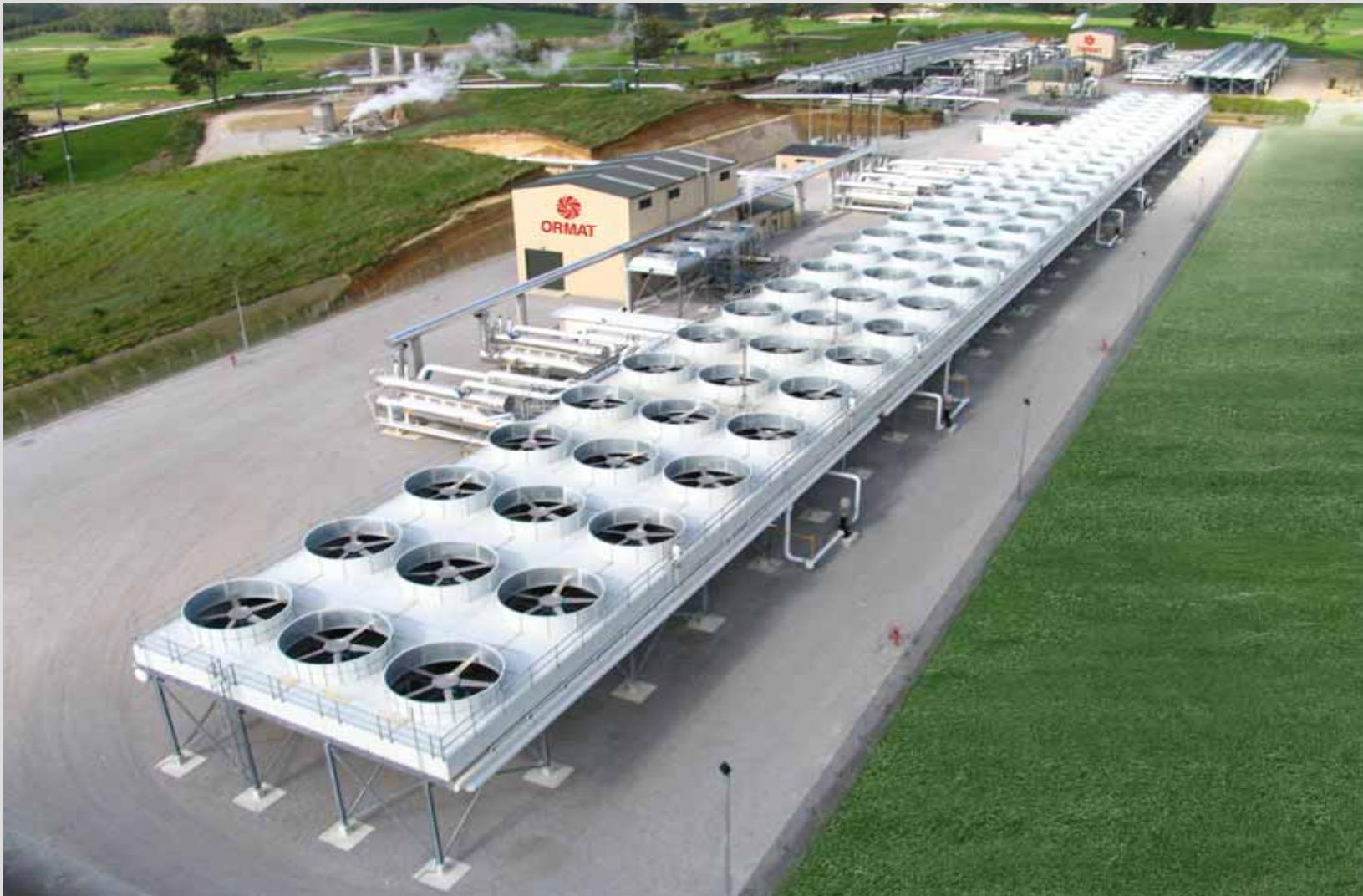
100 MW air cooled geothermal power plant, operating from steam and brine at
