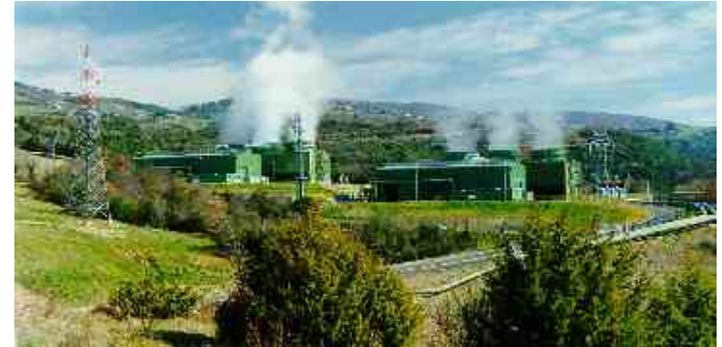
Geothermal power plant
