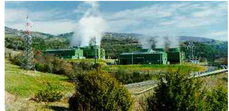
Geothermal power plant
