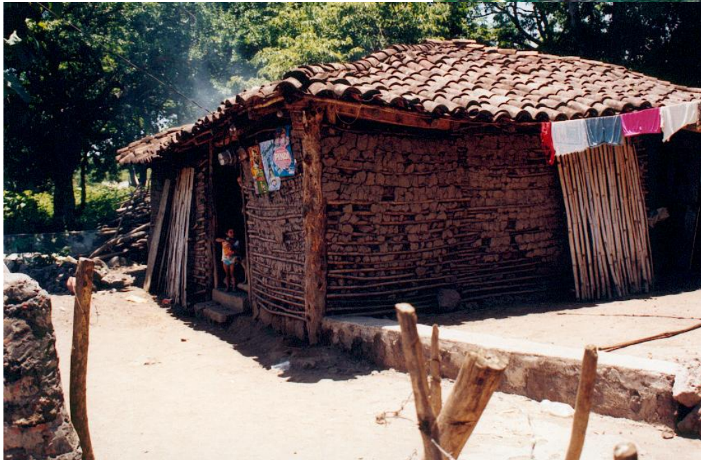
Bahareque housing near TR8A. Note the typical heavy roof on a weak framework.
