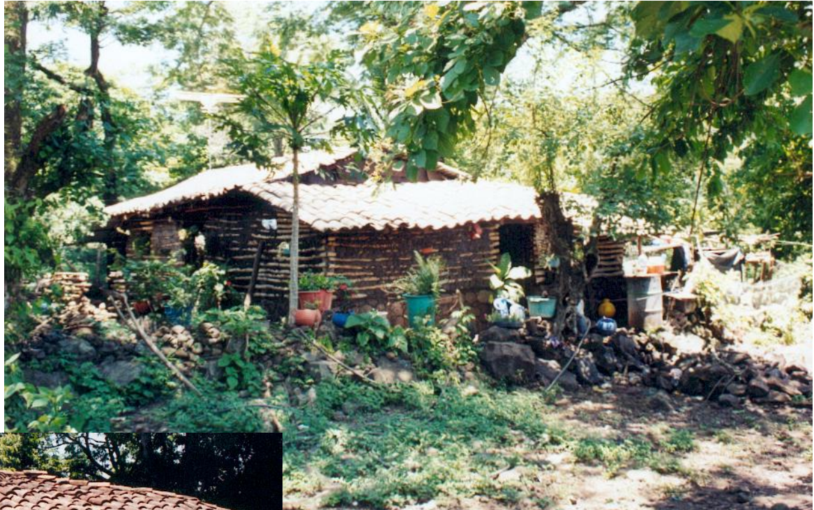
Bahareque housing near TR8A. Note the typical heavy roof on a weak framework.
