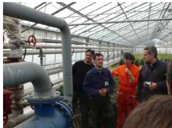
Visiting a greenhouse heated by geothermal energy in the Larderello area.
