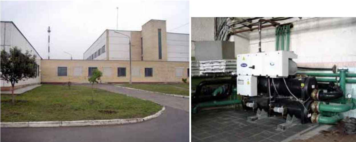
Fig. 3 – A heat pump installation (to the right) based on the utilization of the ground water heat, located in the close vicinity to Minsk and the building (to the left) with a heating supply from this heat pump system. At the background a chimney is shown of the switched off local boiler-house using a natural gas. It is put into operation only when the outdoor air temperature drops below minus 24 °C (photo done by I. Zhidovich).
